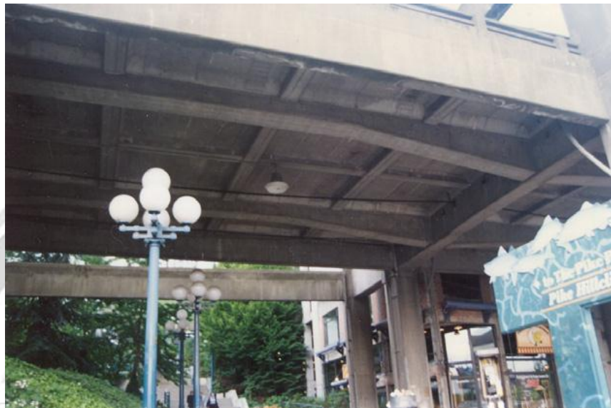
Fig. 1. Urban bridge with RC non-prismatic beams in downtown Seattle [9]
