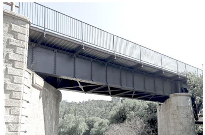
Figure 1 Downstream elevation view of Vilagarcía bridge.
