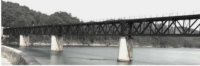
Figure 2 Downstream elevation view of O Vicedo railway bridge.
