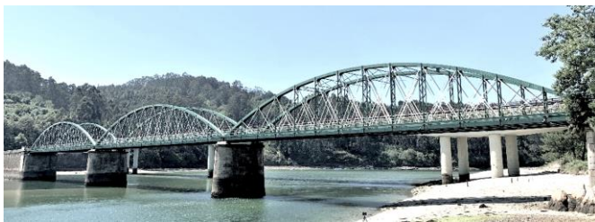
Figure 3 Upstream elevation view of O Barqueiro bridge.
