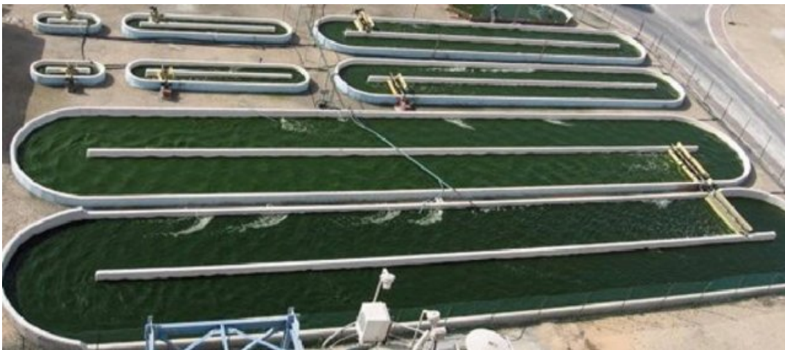
Figure 1: Open-channel raceway ponds in California, U.S. (Source: www.atlanticgreenfuels.com )
