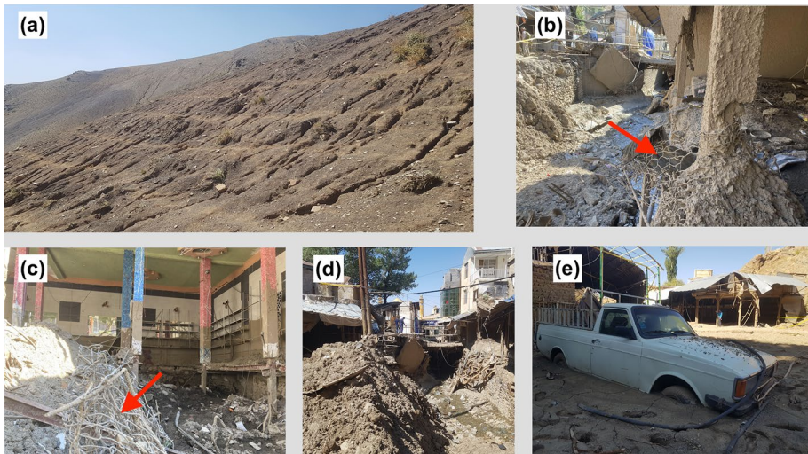
Fig. 4 a Degraded vegetation and intensive slope erosion in an altitude of 2900 m of Emamzadeh Davood upstream. b–e Examples of destruction to infrastructure in Emamzadeh Davood due to the 2022 flood. The remaining of metal nets from gabion check dams around columns of destroyed buildings has been marked with a red arrow in (b) and (c) (Photos credit H. Akhani)
