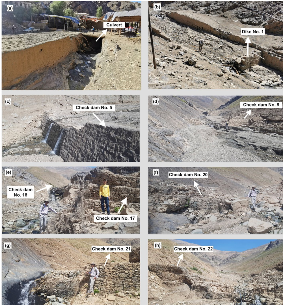
Fig. 3 a–h Exemplary ground photos of check dams and other construction. Photos taken on August 18, 2022. For the location of objects please refer to Fig. 2a (Photos credit H. Akhani)
