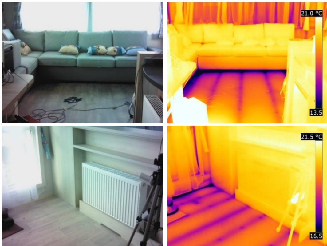
Figure 27 Thermal bridging at the ground floor joists.
