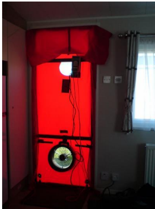
Figure 2 Pressurisation test being undertaken on one of the test caravans.
