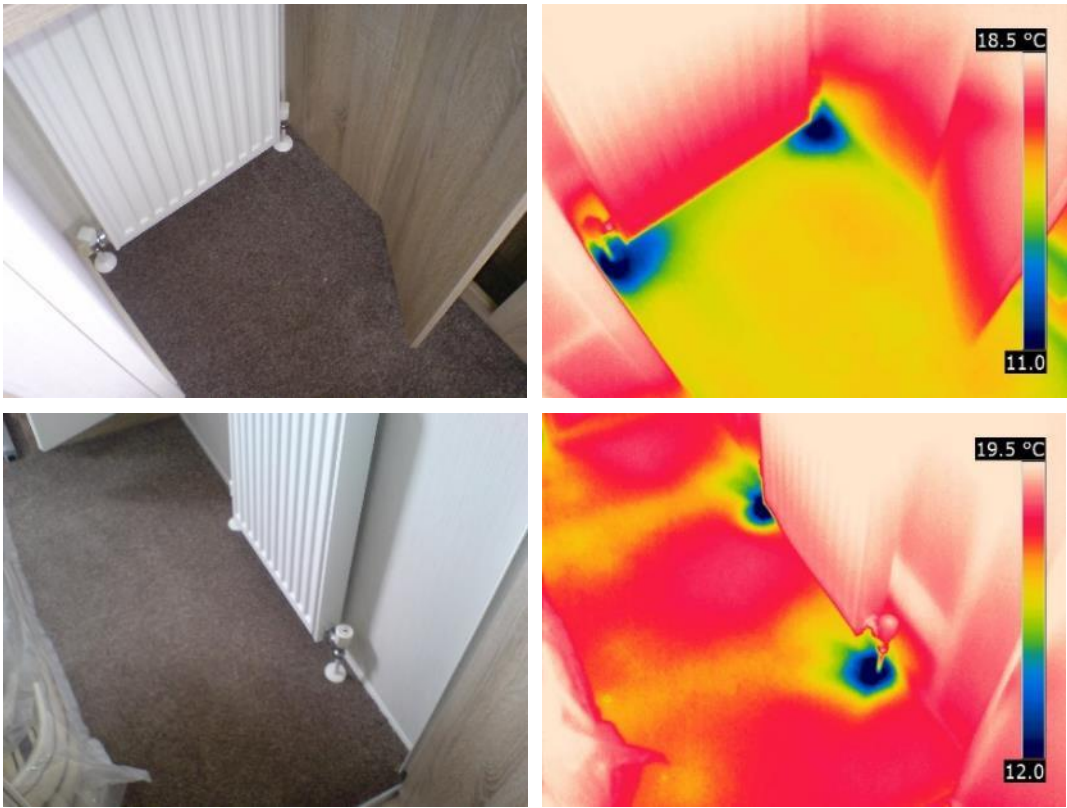
Figure 15 Air leakage around the central heating pipes where they penetrate through the ground floor.
