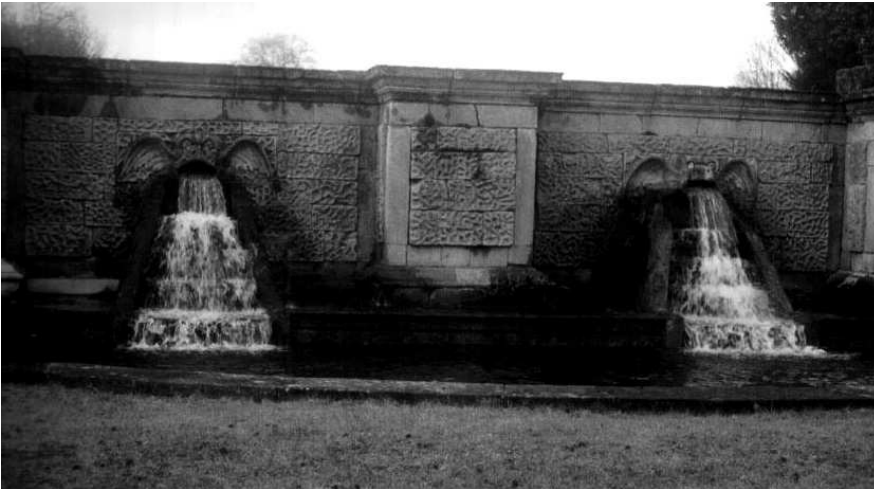
Figure 6. Dragon's mouths at the Obelisk Pond in January 2003 which once supplied water to a long flowing cascade (For most of the year the flow is much less than shown in the figure)
