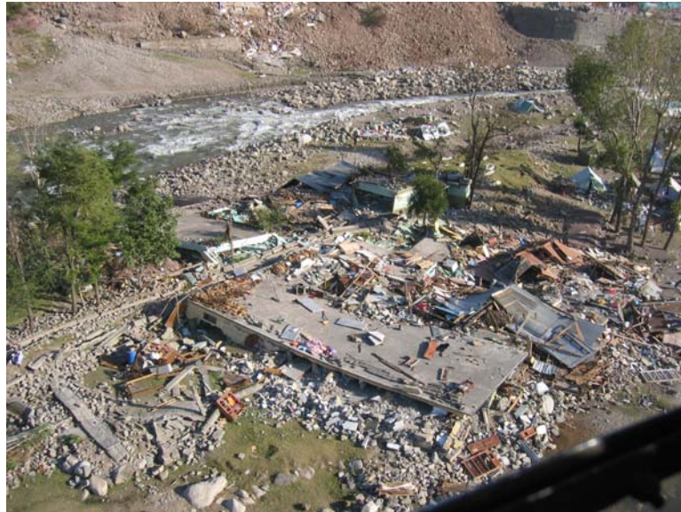
Figure 2.3. Example of a collapsed home in Balakot. Notice the walls have failed and the roof has “pancaked”, crushing the contents of the home. Source: Author.
