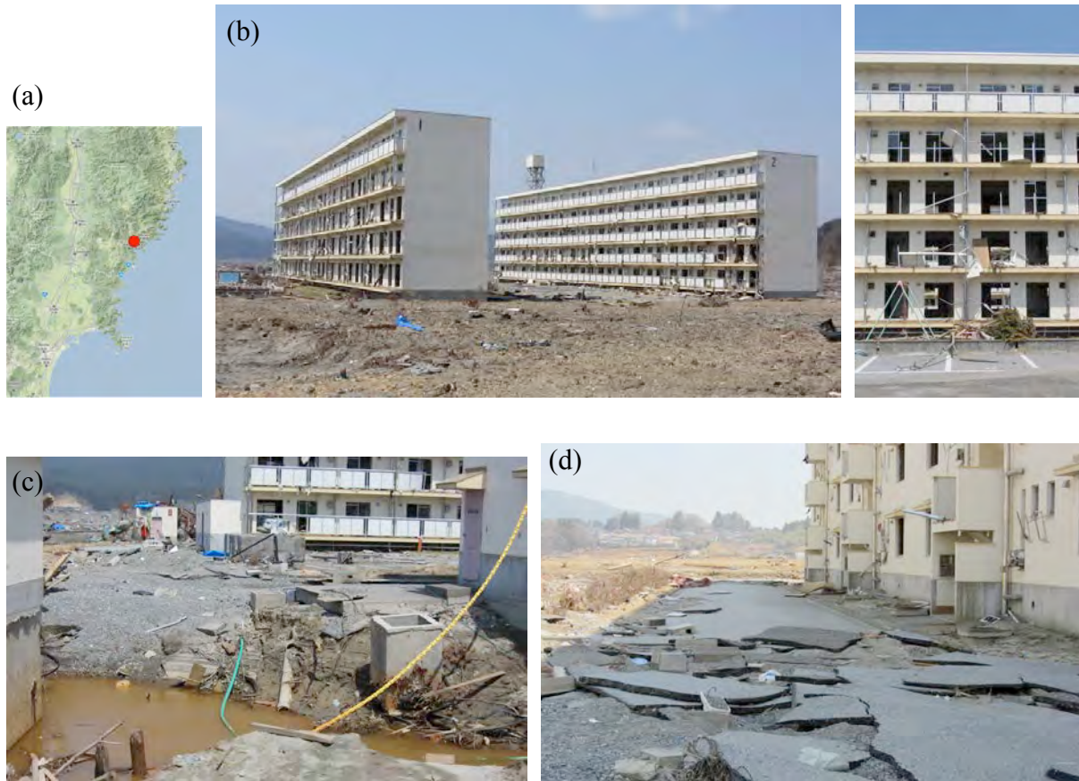
Figure 4. The RC apartment buildings survived in Rikuzen-Takata. The average runup height in the vicinity was 14.2 m. (a) The location of Rikuzen-Takata ( 39^{\circ}00.5'N 141^{\circ}38.3'E ). (b) The tsunami punched through from the front to back doors and windows to create many piercing holes, which must have reduced tsunami forces. (c) A deep scour hole at the side of the first building facing to the sea and (d) the ripped asphalt slabs in the sheltered area behind the first building.
