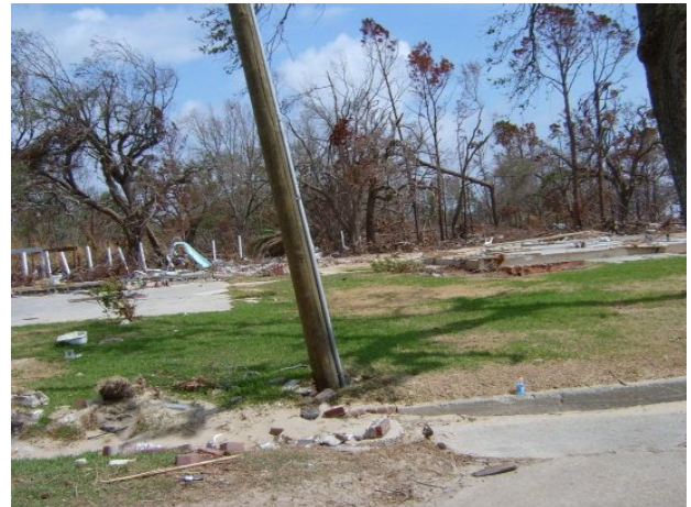
Fig. 1. The foundations of houses in waveland, mississippi, USA following Hurricane Katrina in 2005.
