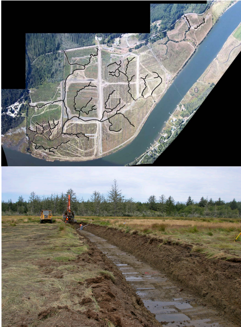
Figure A20. Top: Restored (excavated) marsh channels (black lines). Background is August 2010 aerial by Roy Lowe. Bottom: Newly dug channel form.
