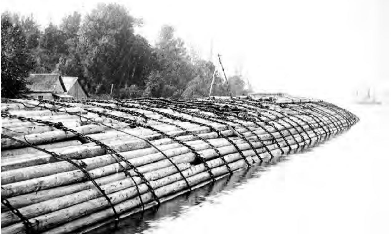
Chains and cables holding together completed Benson raft, Columbia River near Stella, Washington, ca. 1903, by John Fletcher Ford. University of Washington Libraries, Special Collections, J.F. Ford Photograph Collection, box 1, folder 5, item 45, PH Coll 701.45. digital.lib.washington.edu/findingaids/view?docId=FordJFPHColl701.xml .
