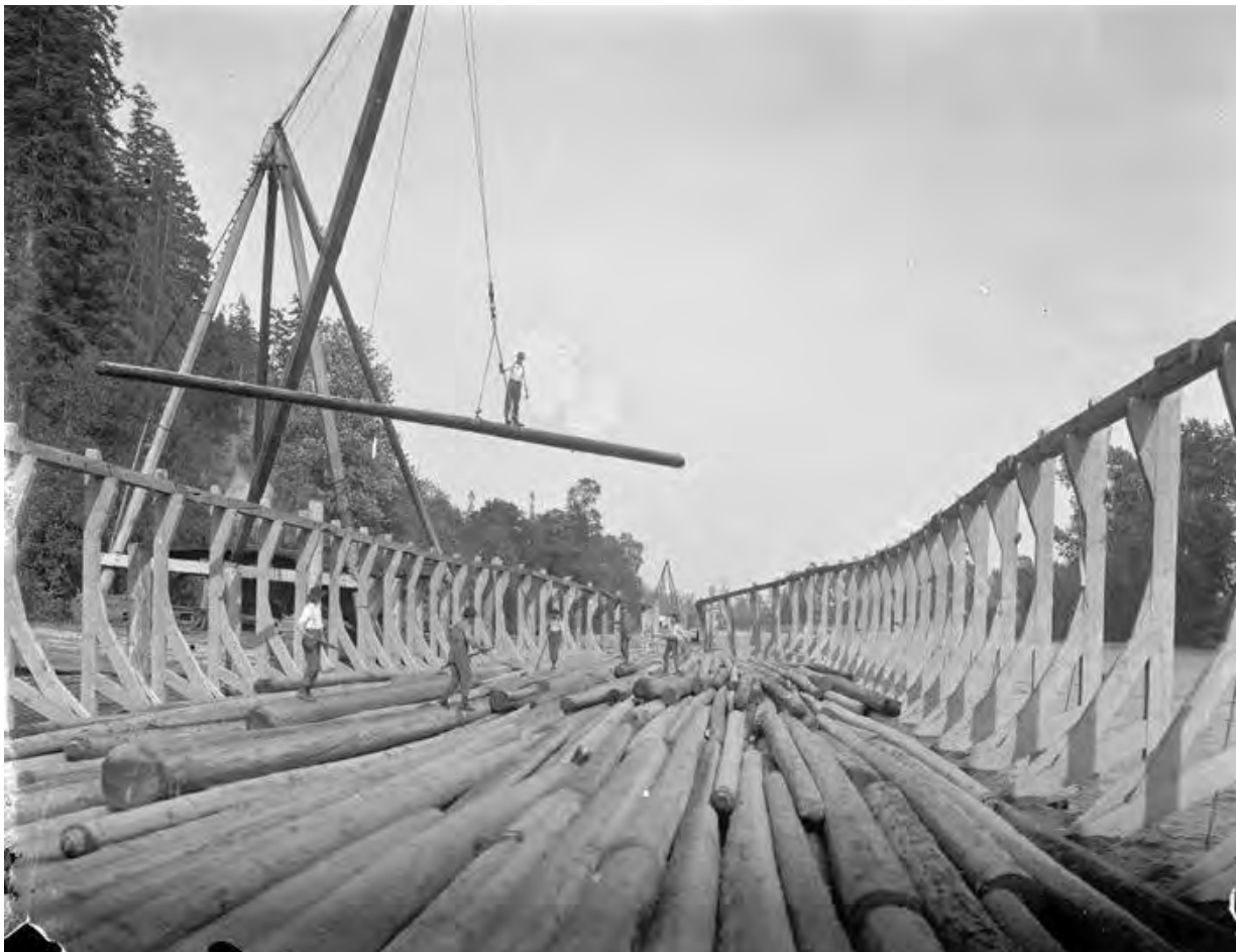
Crew arranging logs inside cradle, Columbia River near Stella, Washington, ca. 1903, by John Fletcher Ford. University of Washington Libraries, Special Collections, J.F. Ford Photograph Collection, box 1, folder 5, item 39, PH Coll 701.39. digital.lib.washington.edu/findingaids/view?docId=FordJFPHColl701.xml .
