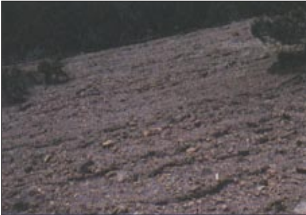
Photo 19.— This site has been allowed to deteriorate perhaps beyond its ability to recover. Nevertheless, it is critically important to control juniper and scatter slash if only to slow sediment movement.
