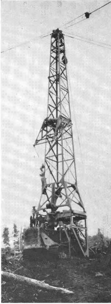
Figure 7. Tractor-mounted tower used by the Crown Zellerbach Corporation in Clatsop County, Oregon. The tower is hinged in the center and at the point of attachment to the tractor. It is lowered when the unit makes a long move.
