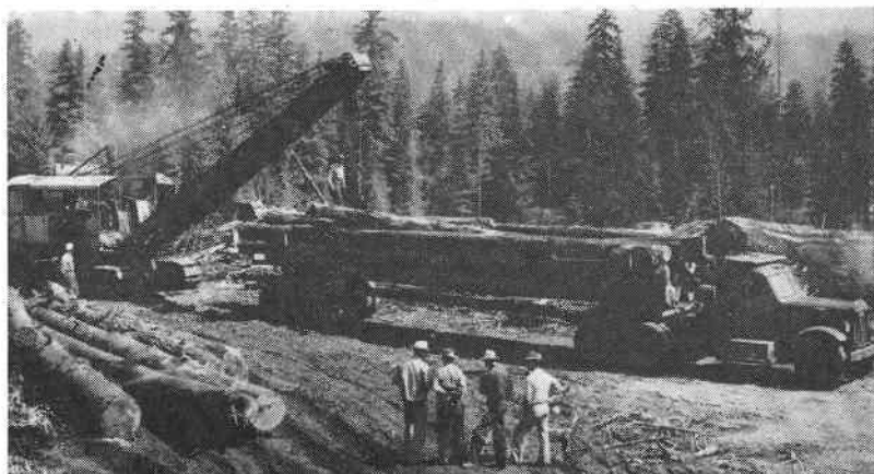
Figure 15. Conventional log truck and trailer equipped with 36-inch stakes to facilitate the loading of salvaged logs.
