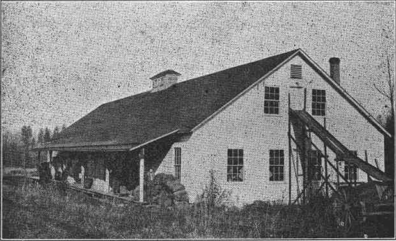
Fig. 12. Packing House of A. P. Paasch, Hood River, Oregon. A Medium Priced Packing and Storage House. Notice the Ventilator and the Chute for Sending Boxes from the Upper Floors.
