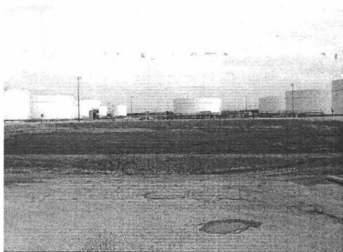
Photograph 1 Tank Farm at the Kansas City Site, Kansas City, KS.
