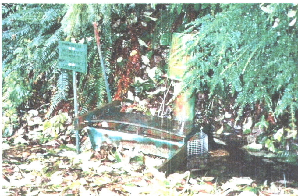
Figure 4. Flume installation at road segment 15-8-1.2.
