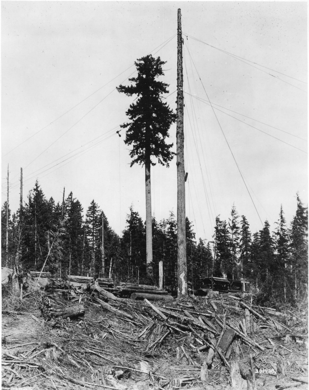
331199 SPAR TREE AND RIGGING FOR ELECTRIC LOGGING OPERATIONS. SNOQUALMIE, FALLS LUMBER COMPANY, SNOQUALMIE FALLS, WASHINGTON.
