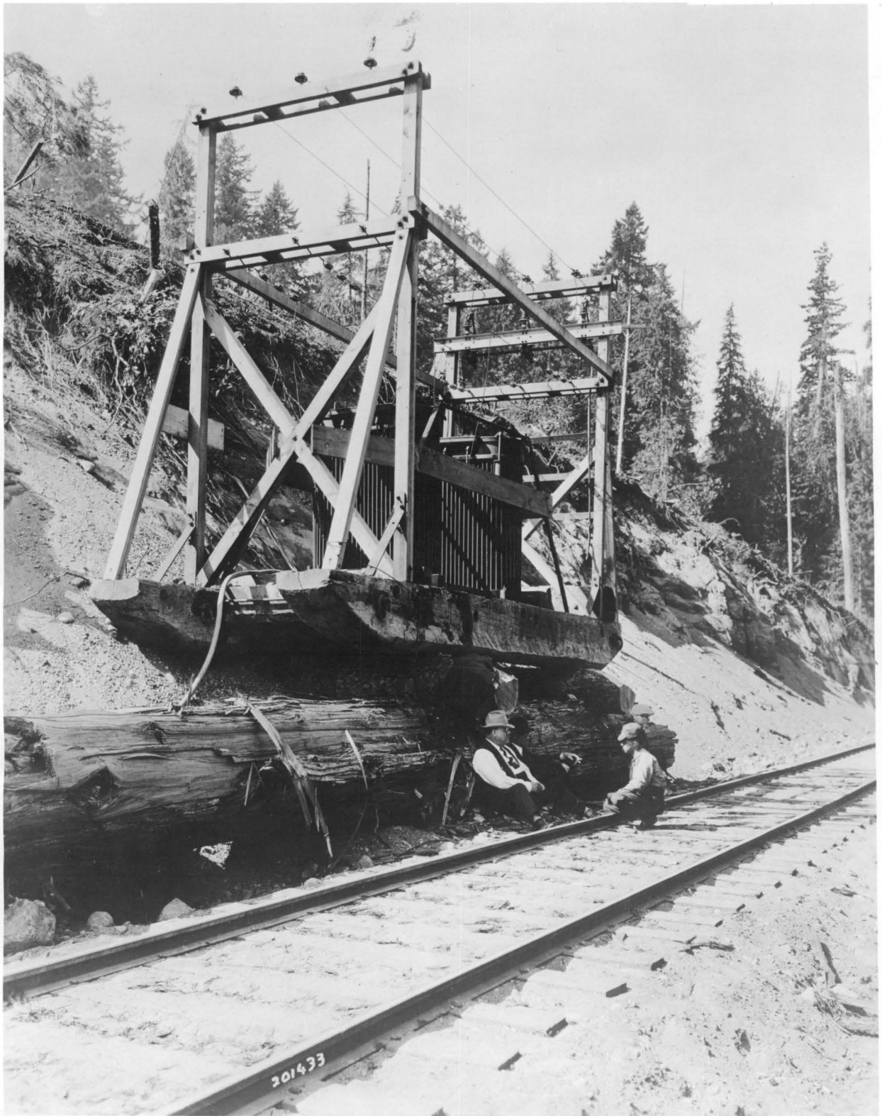
331198 PORTABLE TRANSFORMER SUBSTATION 2-250KV-A- 3 PHASE-13200/600 VOLT TRANSFORMERS.
