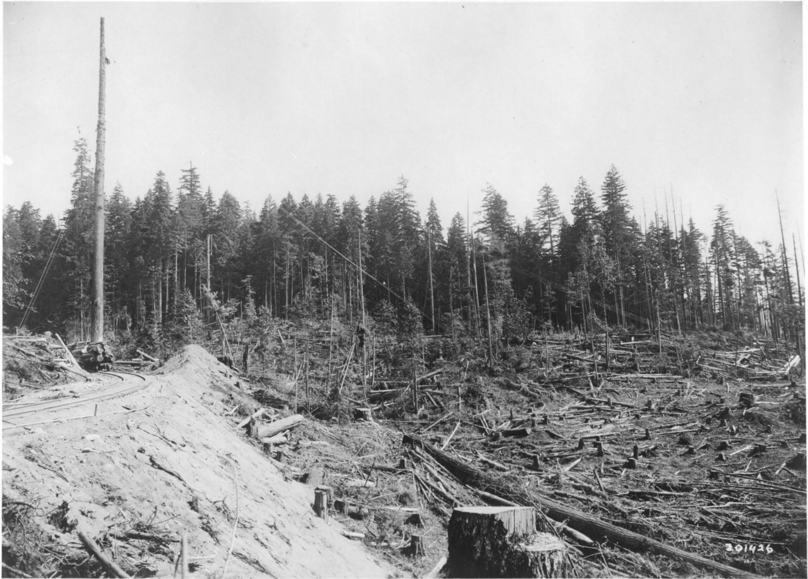
331200 SPAR TREE AND RIGGING FOR ELECTRIC LOGGING OPERATIONS, SNOQUALMIE FALLS LUMBER COMPANY, SNOQUALMIE FALLS, WASHINGTON.
