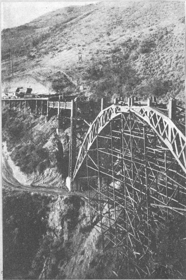
Fig. 7- Dolan Creek Arch Bridge
