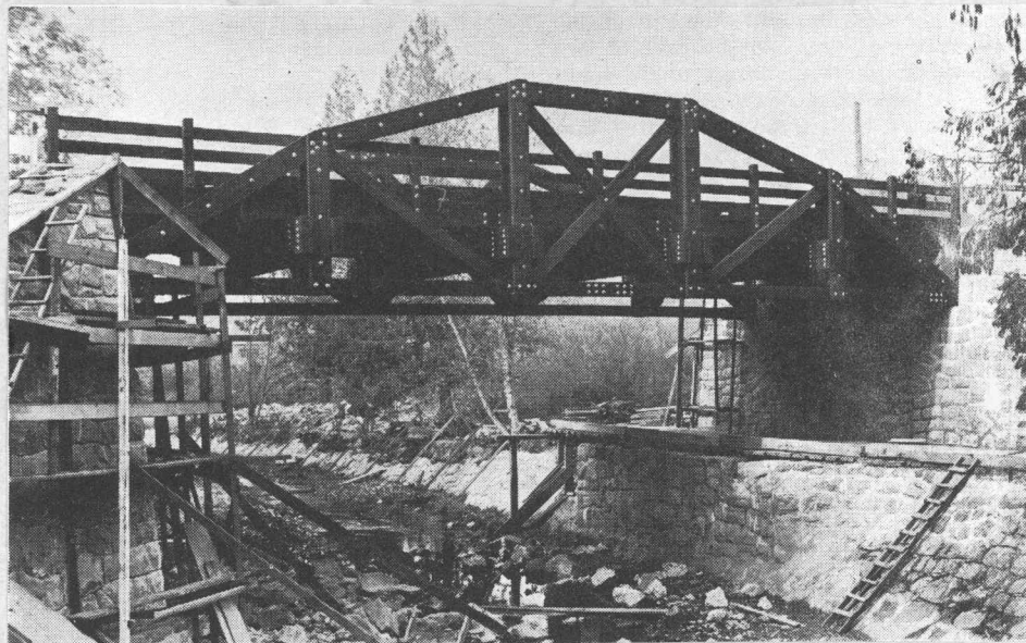
Fig. 6- Johnson Creek Bridge
