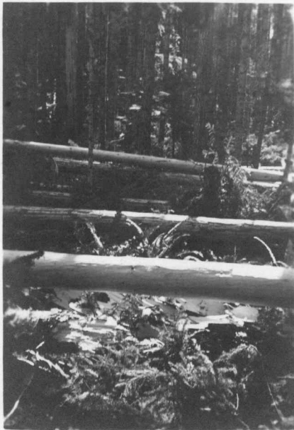
Piling felled and peeled.
