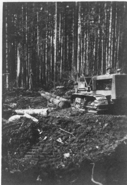
Cat skidding peeled piling from the woods to the landing.
