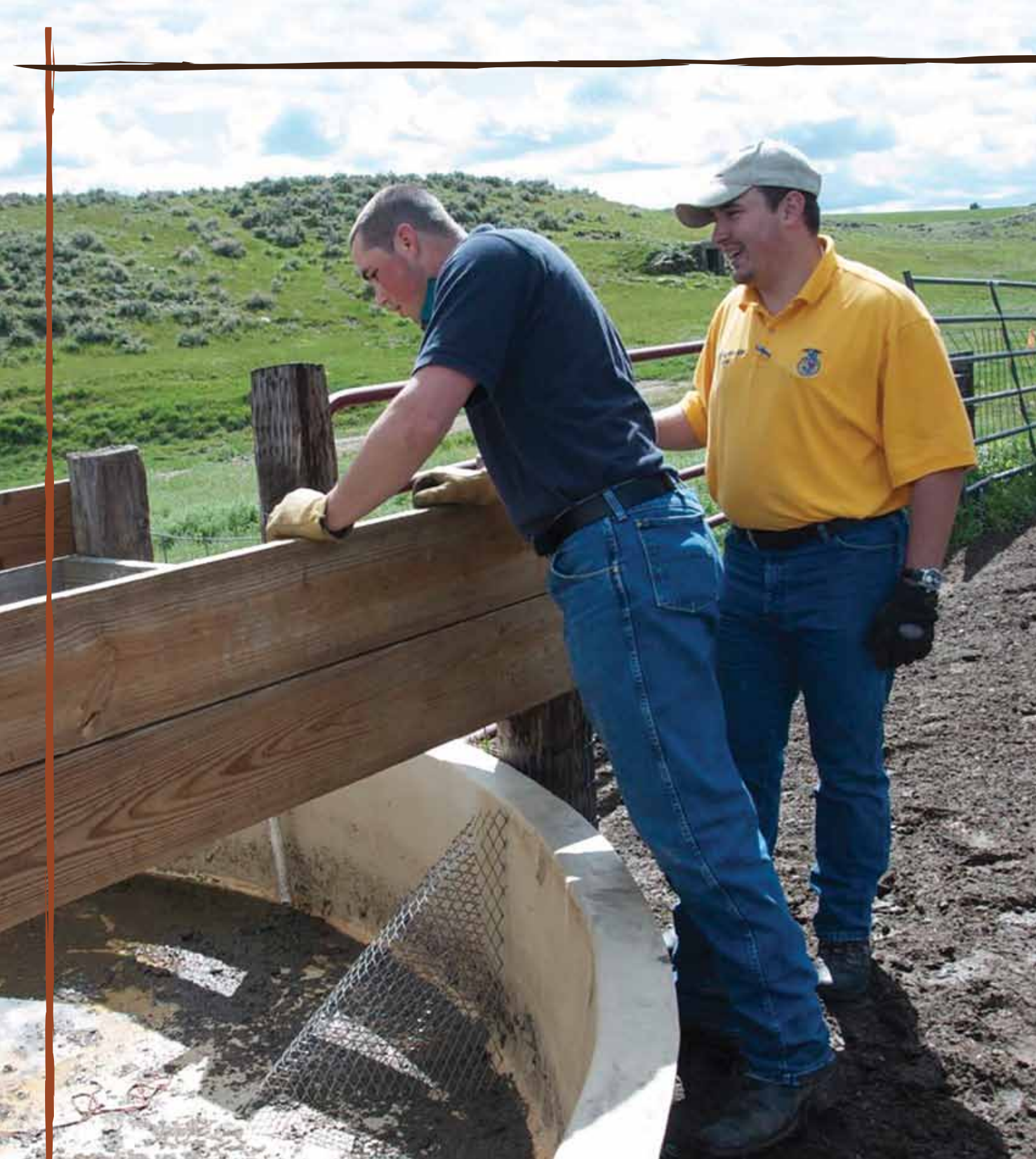
Volunteers retrofit livestock water tanks to add escape ramps for sage grouse and other wildlife.
