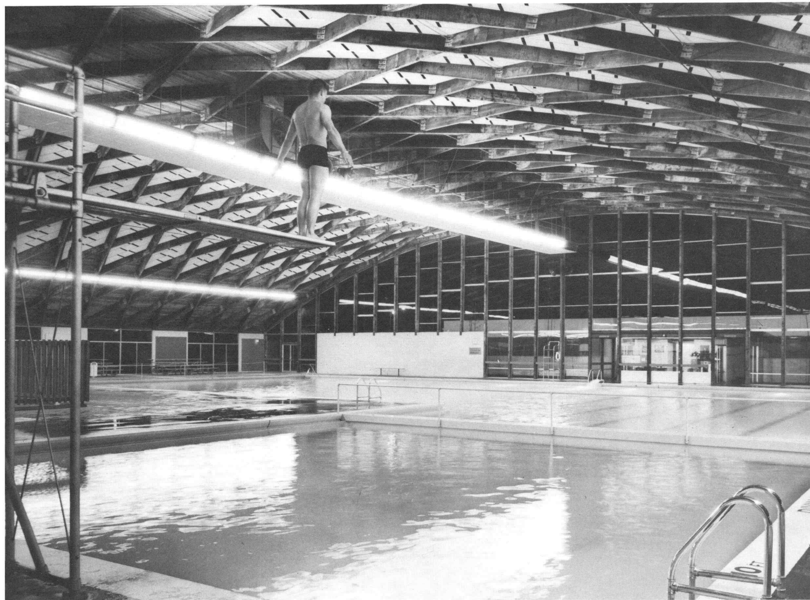
The roof structure over the Willamalane Park & Recreation District swimming pool, with a span of 173 feet, was the largest wood lamella structure ever built (1961). The roof lamella used 60,000 board feet and the roof decking 67,000 board feet. (Photo by Willamalane Park & Recreation District, Springfield.)
