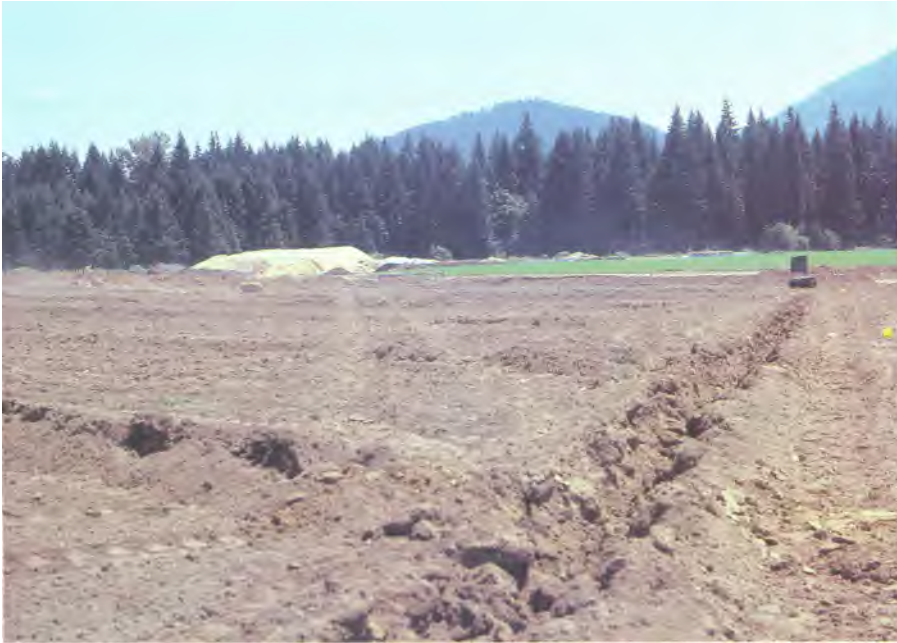
Figure 33-7. Water management is sometimes difficult in Pacific Northwest nurseries because of high rainfall and heavy soils. Tiling areas prior to sowing helps ensure good drainage.
