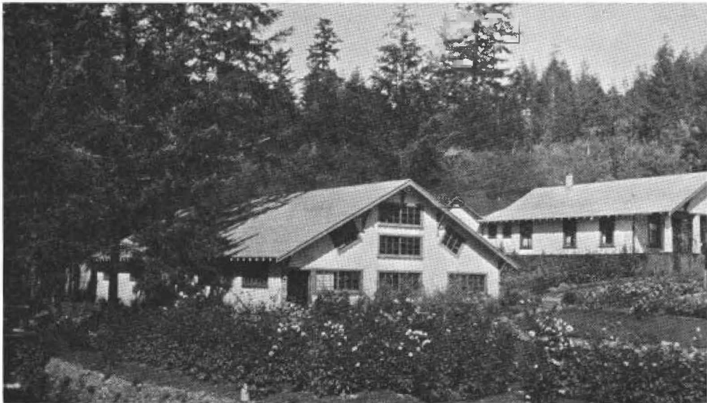
UMPQUA RIVER HATCHERY BUILDING AND DWELLING, ROCK CREEK, DOUGLAS COUNTY
