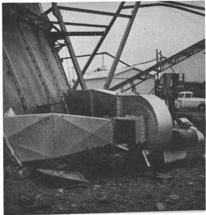
Figure 12. A combination forced-overfire-air and gas-recirculation system.
