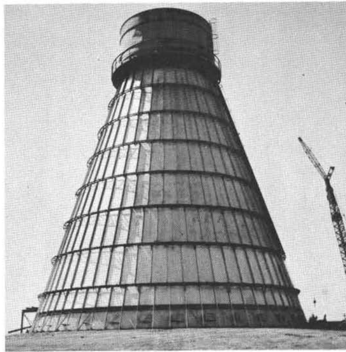
Figure 14. A water-wash scrubber on a new burner at Memphis, Tennessee.
