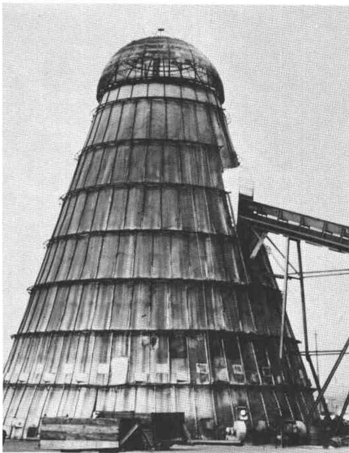
Figure 5. A 67-foot burner near Medford, Oregon, operating with bark and sawdust.
