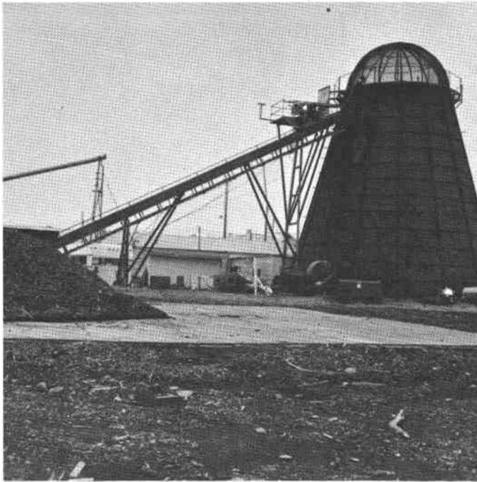
Figure 17. Wigwam burner test site.
