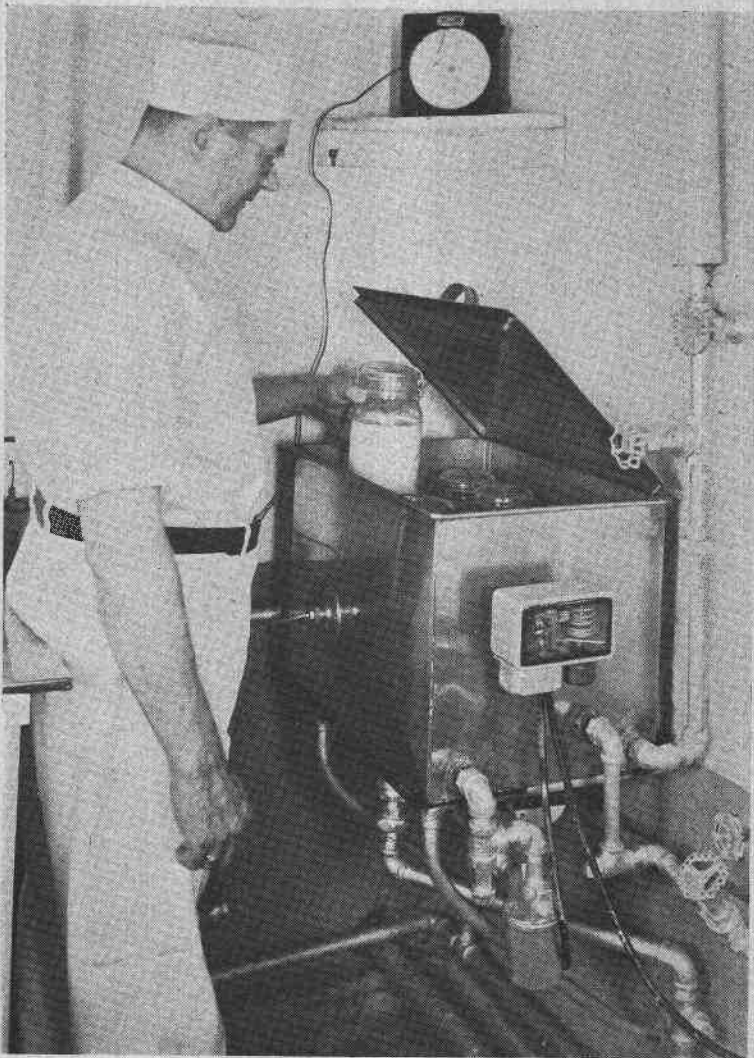
Figure 3. PREPARING MOTHER CULTURE UNDER CONTROLLED CONDITIONS.
