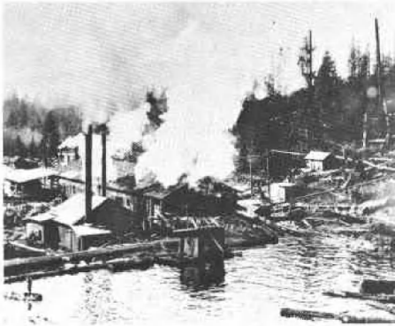
Figure 7. Early sawmills used steam produced from wood fuel as a power supply for the mill.
