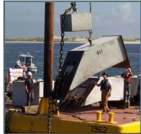
Figure 13 Enhanced Deadweight Anchor
