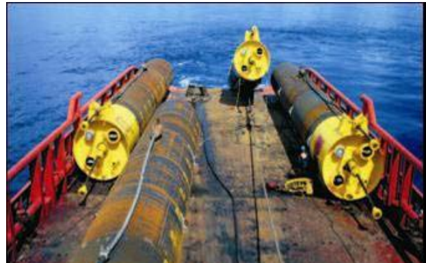
Figure 17 Multiple Suction Piles Installed from Single Vessel
