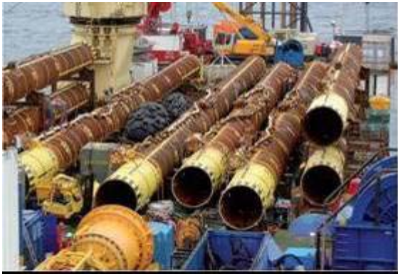
Figure 16 Multiple Mooring Piles Loaded for Transport
