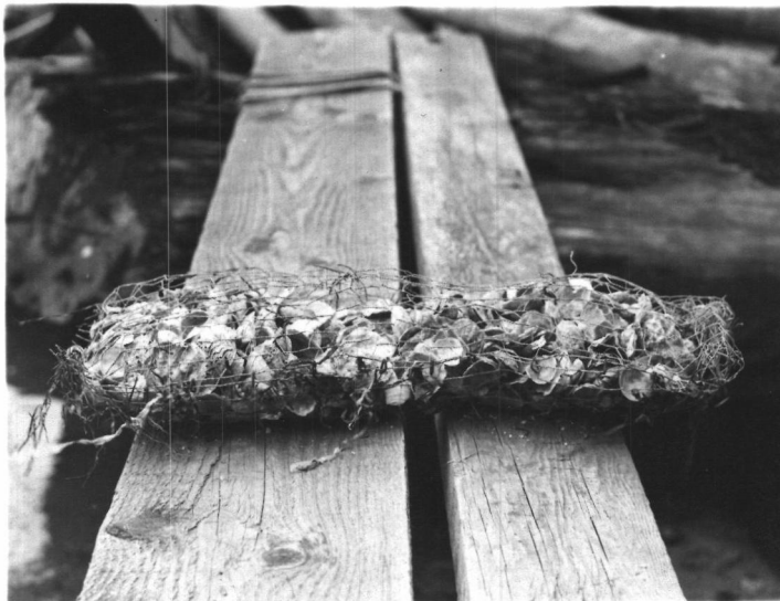
Wire bag filled with native oyster shells.
