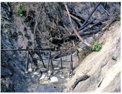
Figure 35. Severe fires that consume protective vegetative cover and organic layers of forest soil can lead to erosion, land slides, debris flows, and other adverse effects. This scene shows a debris rack installed in a stream to impede the movement of woody material downstream.
