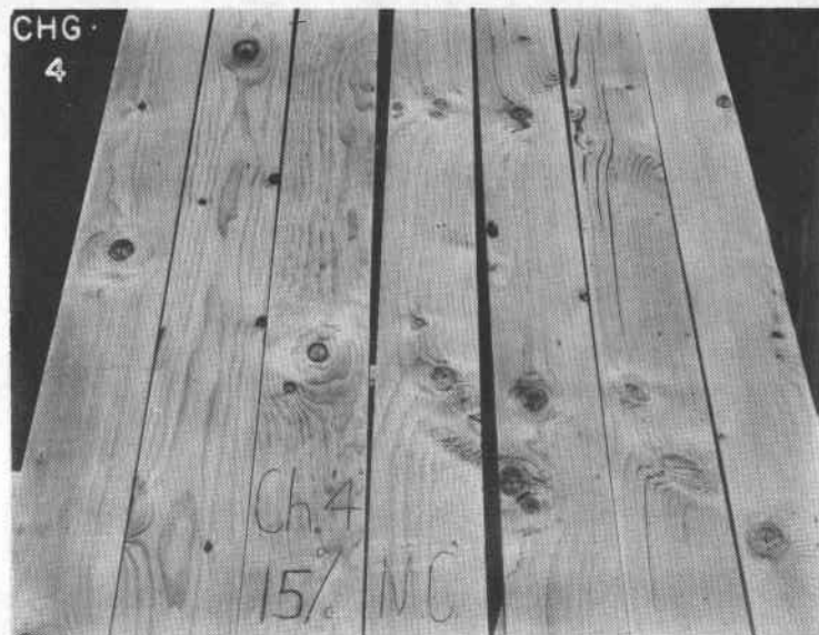
FIGURE 17. CONDITION OF KNOTS AFTER SURFACING: CHARGE 4.
