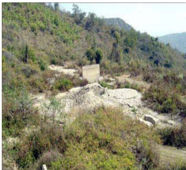
Figure 3.2. Abandoned Hundung Cement Factory
