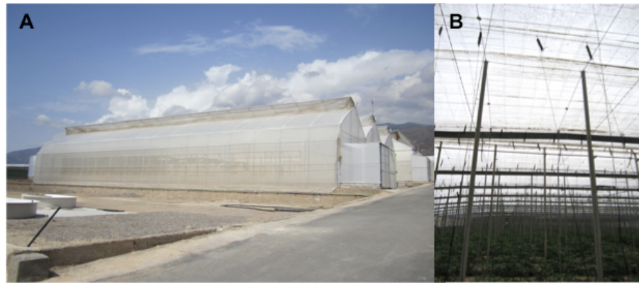
Figure 10. Typical parral or Almería -type greenhouses used for tomato production. (A) These greenhouse structures are covered with polyethylene plastic film ( Photograph taken 09/20/2010 at Las Palmerillas – Cajamar Experimental Station, Almería ). (B) The polyethylene material is held up by braids, cords, and wires attached to metal poles to create the house-shaped structure ( Photograph taken by Theresa T. Nguyen on 9/20/2010 at Cooperativa Agrícola San Isidro (CASI), Almería ).
