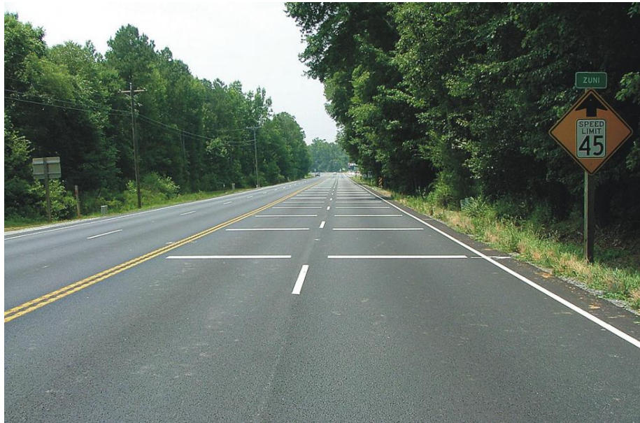
Figure A.7: Full Width Transverse Bars Source: Arnold & Lantz, 2007
