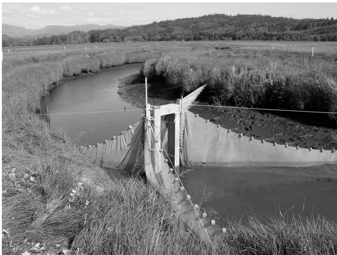
Figure 3.2. Antenna 1 installed in study channel at a moderately low tide.
