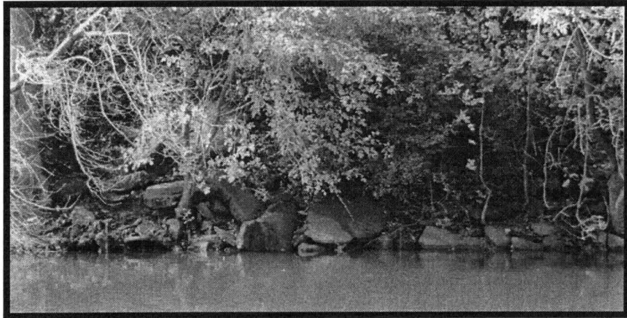
Figure 37. Concrete and debris at the end of Monroe Avenue.
