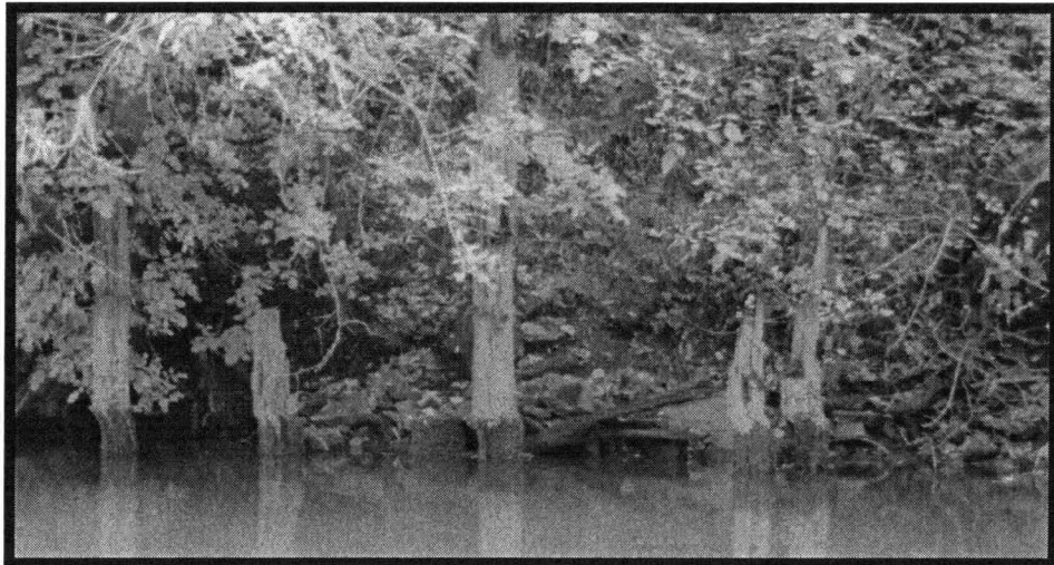
Figure 36. Wooden pilings in the Willamette River north of Jackson Avenue.
