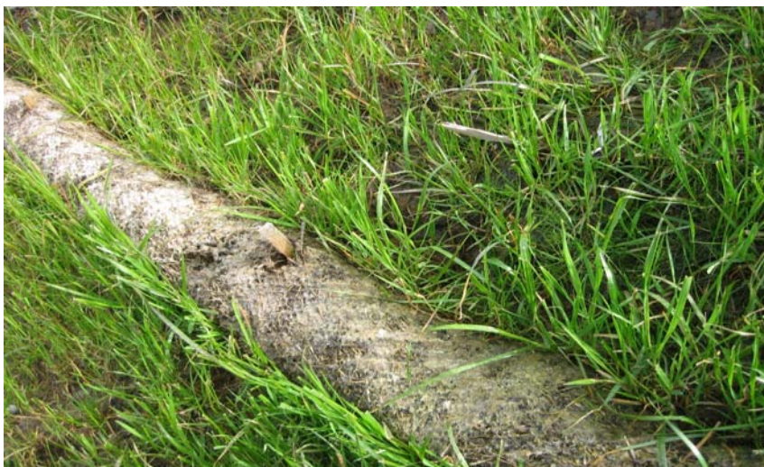
Figure 6. Example of straw wattle placement on-site
