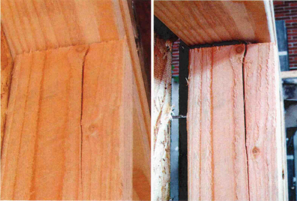
Fig. C3. Split center stud from the 115-ksi wall before (left) after (right).
