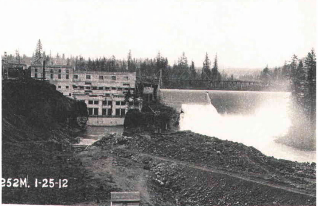
Figure 4.13 Spoil pile below River Mill Dam 2003 and 1912.
