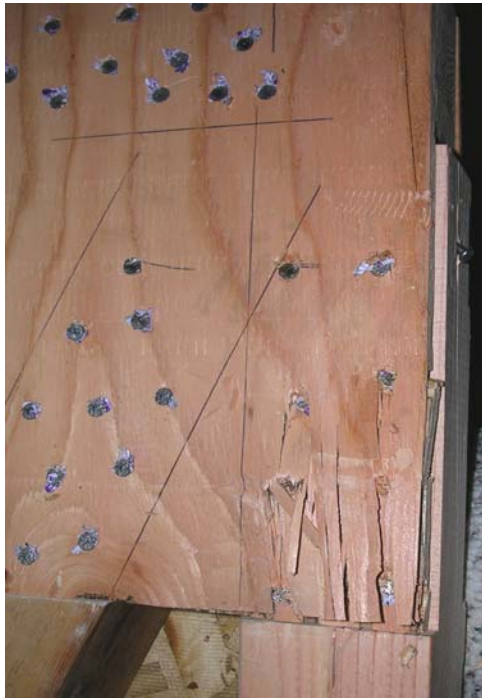
Fig. B21. Plywood gusset plate failure at top corner of wall.
