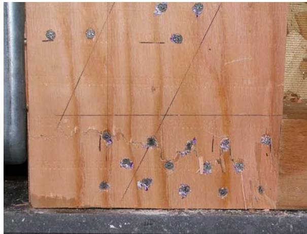
Fig. 3.8. Type 3 shearwall gusset plate failure.
