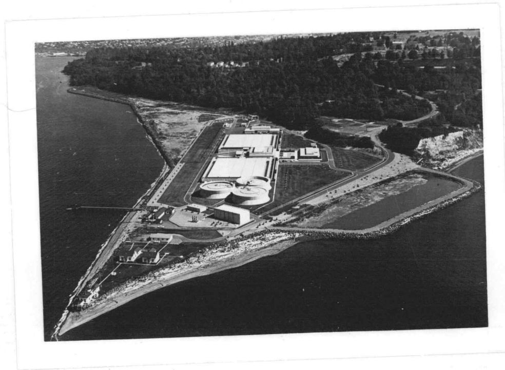
Figure 2. West Point Sewage Treatment Plant. Shilshole Bay is to the left, Fort Lawton is in the background (trees).
