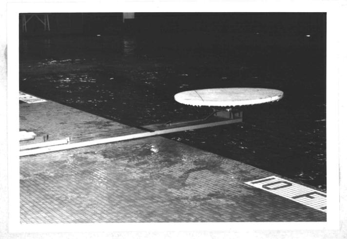
disc's mounting. This design allowed the disc to be rotated freely in either direction and the box to be tipped to a 290° angle. The surface of the disc was two feet above the water surface and was three feet from the pool edge.
