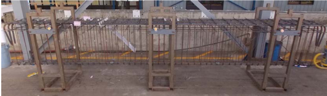
Figure 3.13 – Finished rebar cage
