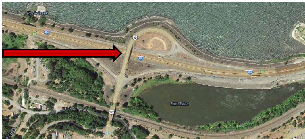
Figure F.1 – Mosier Bridge location over I-84 (Google Maps, 2014)
