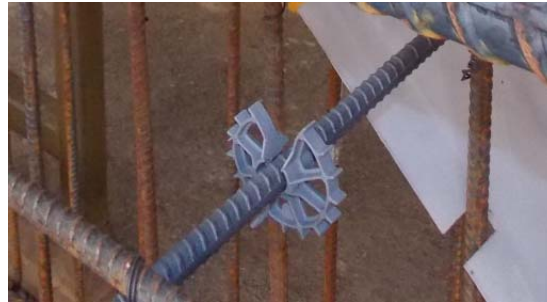
Figure 3.14 – Chair used to ensure cover concrete
