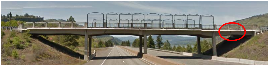
Figure F.3 – Elevation photograph of Mosier Bridge (Google Maps, 2014)
