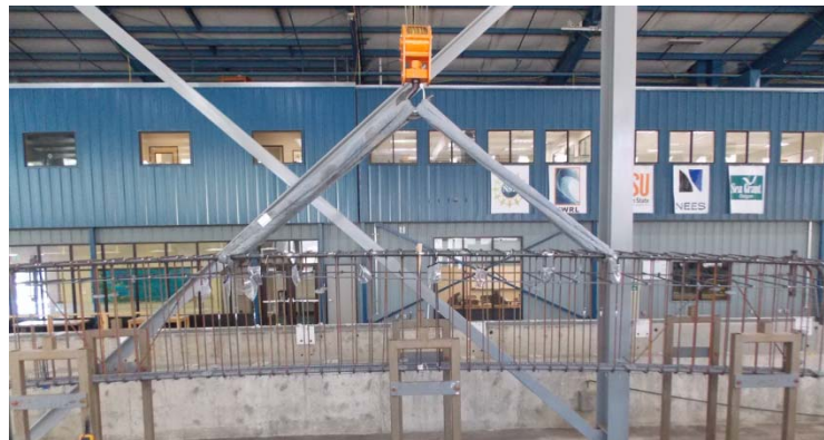
Figure 3.16 – Typical cage lifting process
