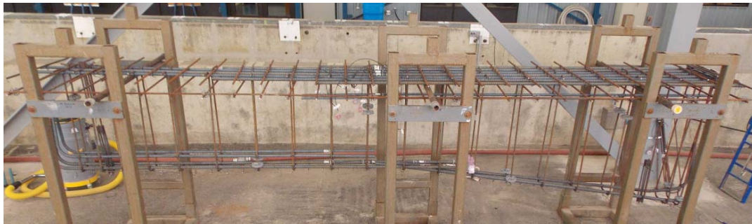
Figure F.19 – Finished rebar cage
