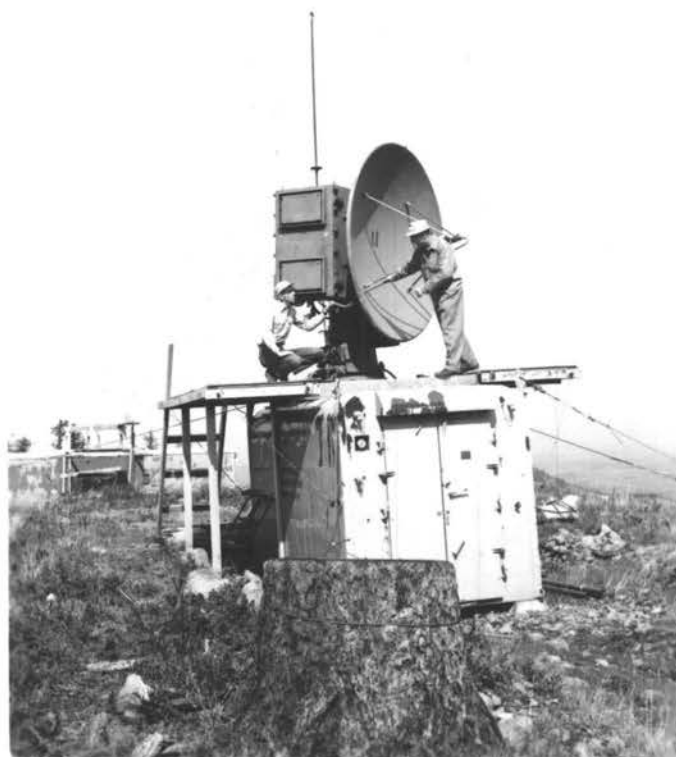
Plate 1. The AN/CPS-9 Weather Radar Antenna.
