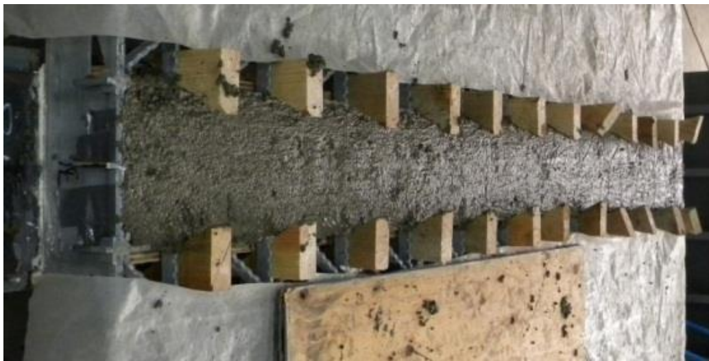
Figure 4.29 Concrete poured flush to top of open grid panel
