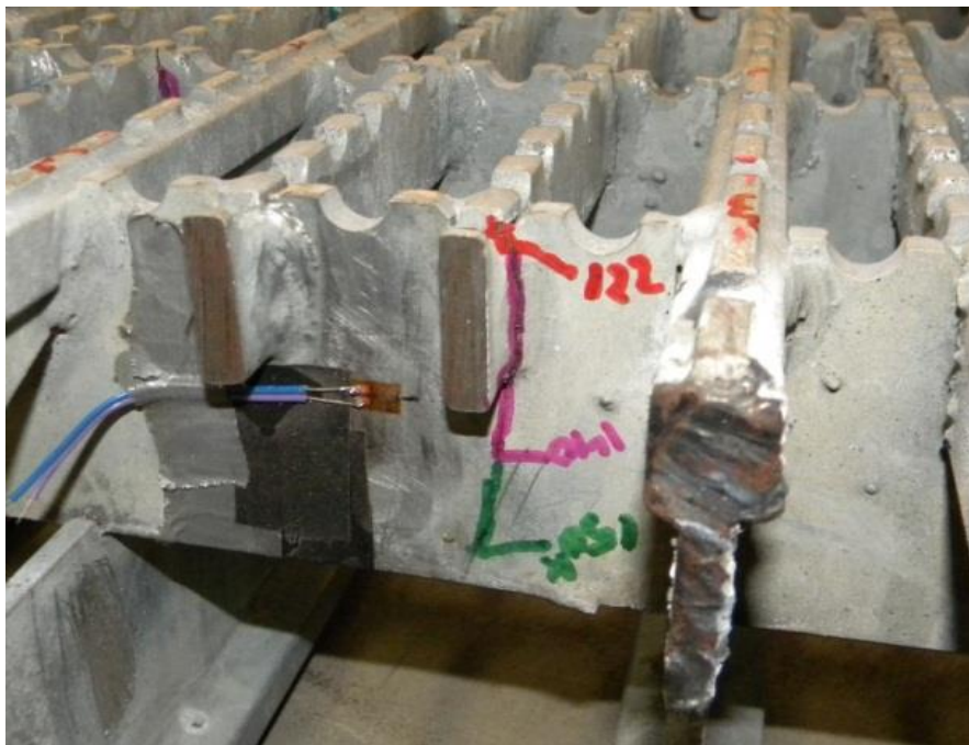
Figure 5.29: 'F' crack initiation from fillet weld
