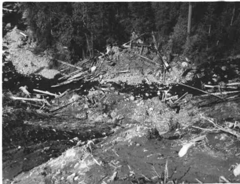
Figure 5. Landslide into Lookout Creek from Road in Unit 1C.
