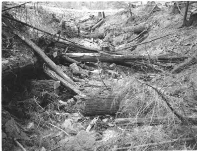
Figure 7. Road Culvert in Tributary 1 in Unit 1C.
