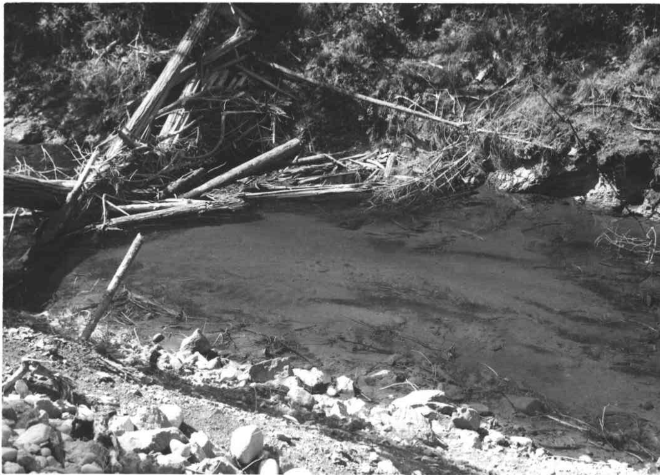
Figure 4. Artificial Pool in Lookout Creek Resulting from Road Construction.
