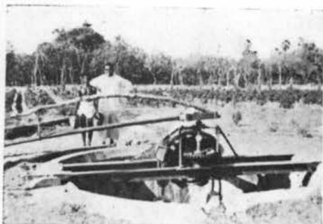
PHOTO 1.—Bullock operated water lift on well.
