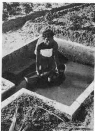
PHOTO 3.—Lined pond for irrigation.
