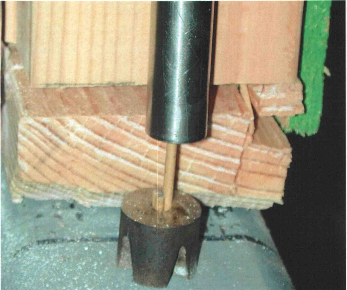
Figure 3. Splitting of sill plate caused by tension perpendicular to the grain
