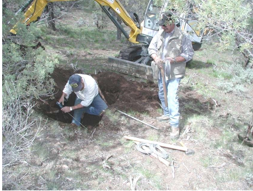
Figure 9. Installation of soil moisture probes
