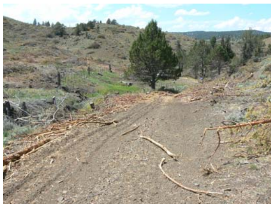
This road was used as a skid trail. Just days before the storm, road condition was soft, with several inches of loose soil on top.
