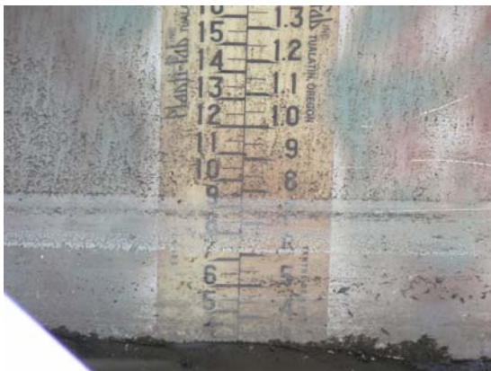
Staff gauge in Jensen flume showed that actual flow may have been as high as 22.86 cm (9 inches). The bottom of the photo shows the height of mud in the flume.
