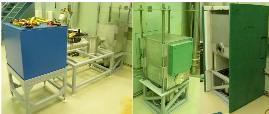
Figure 4-17: Shutter and Beam-stop during installation
