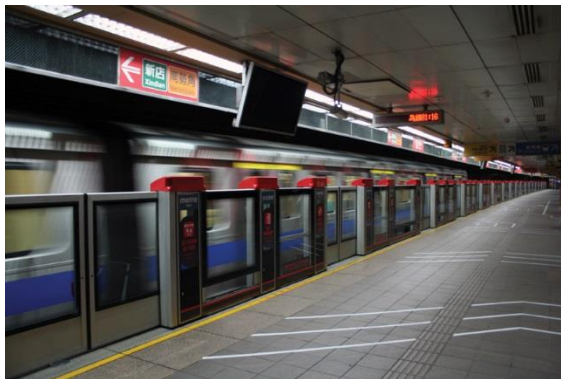
Figure 5: Half Height Platform Screen Doors on Taipei Metro.
