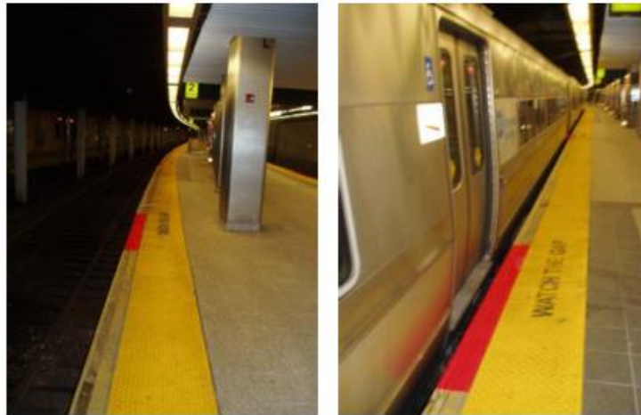
Figure 11: "Watch the Gap" and Red Painted Warning Markings on Long Island Platform (15)
