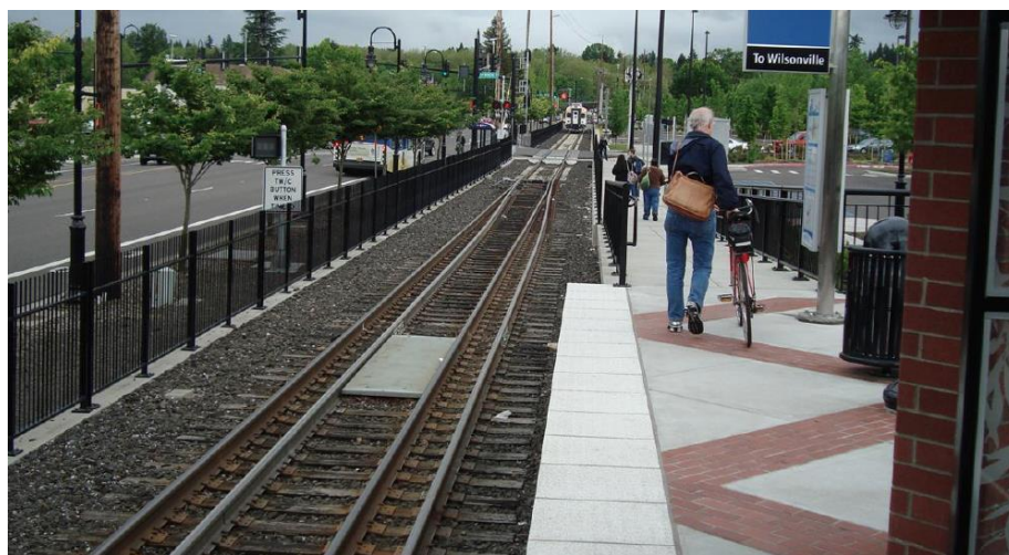
Figure 1: Gauntlet Track at Station in Portland, OR (Ken Kirse).
