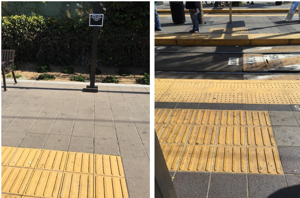
Figure 32: Door Location Bars and Sign for Low Vision and Blind Passengers (San Diego MTS)
