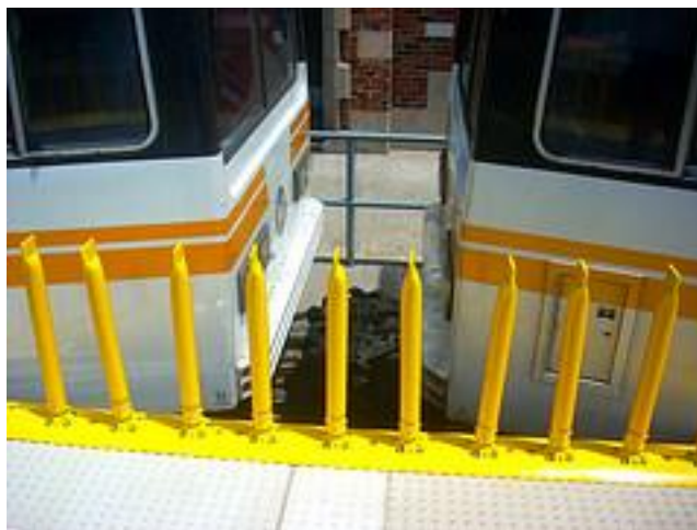
Figure 2: Bollard Between Car Barrier in Los Angeles, CA.
