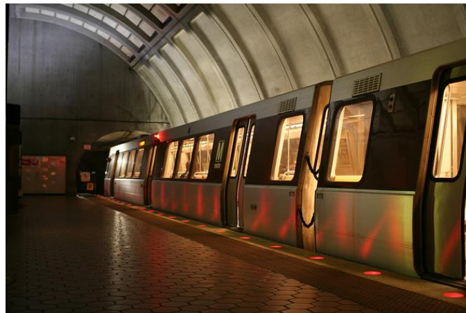
Figure 3: Platform Edge Warning Light Treatment on Washington D.C. METRO (WMATA)
