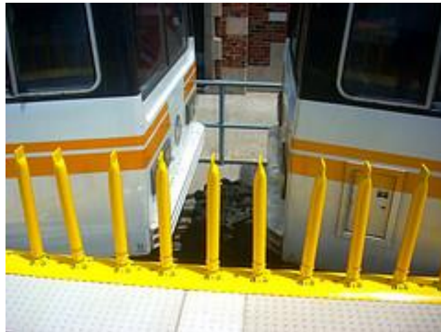
Figure 8: Bollard Between Car Barrier in Los Angeles, CA, USA
