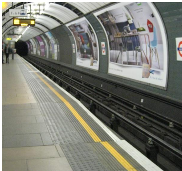
Figure 18: Partially Raised Platform at the London Underground Vauxhall Station
