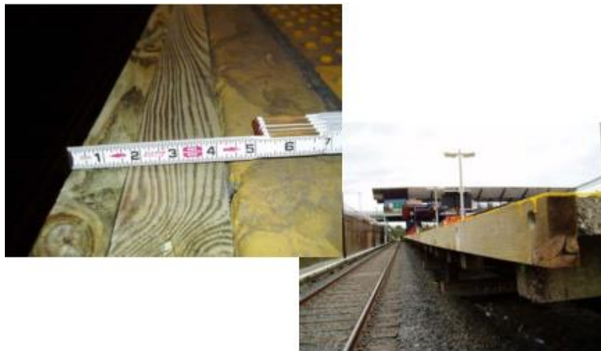
Figure 2: Wooden Edge Boards Installed on Platforms (15)
