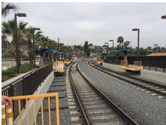
Figure 35: Platform Edge Fencing and Geometric Stabilization (NCTD)
