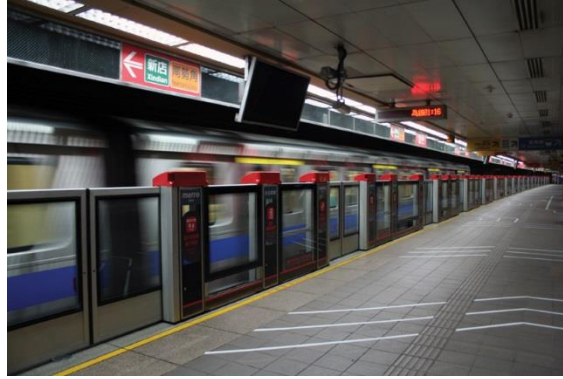
Figure 6: Half height platform edge doors on Taipei Metro
