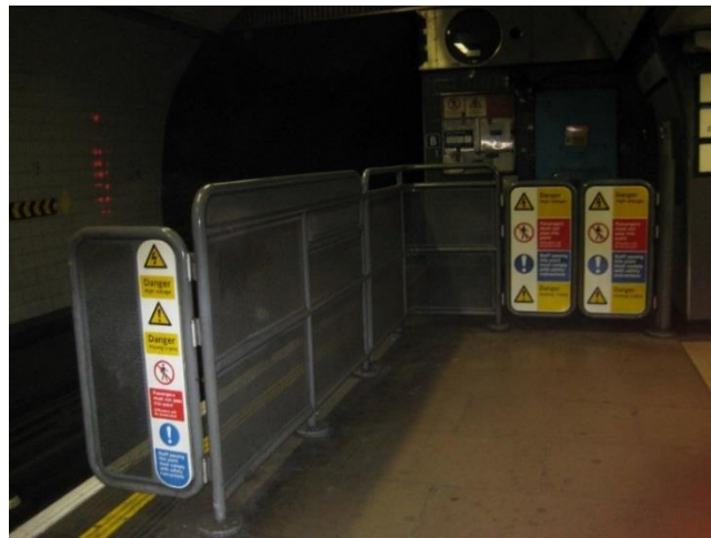
Figure 21: Barriers to Reduce Passenger Intrusion at the End of the Platform
