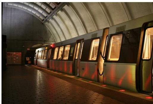
Figure 4: Edge Warning Light Treatment on Washington D.C. Metro.
