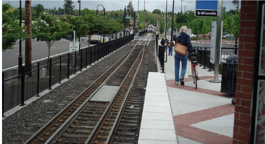
Figure 12: Gauntlet Track at WES commuter rail station in Portland, OR (16)
